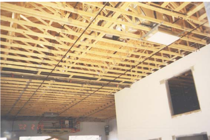
Example of Conventional Construction Wood Roof Trusses
