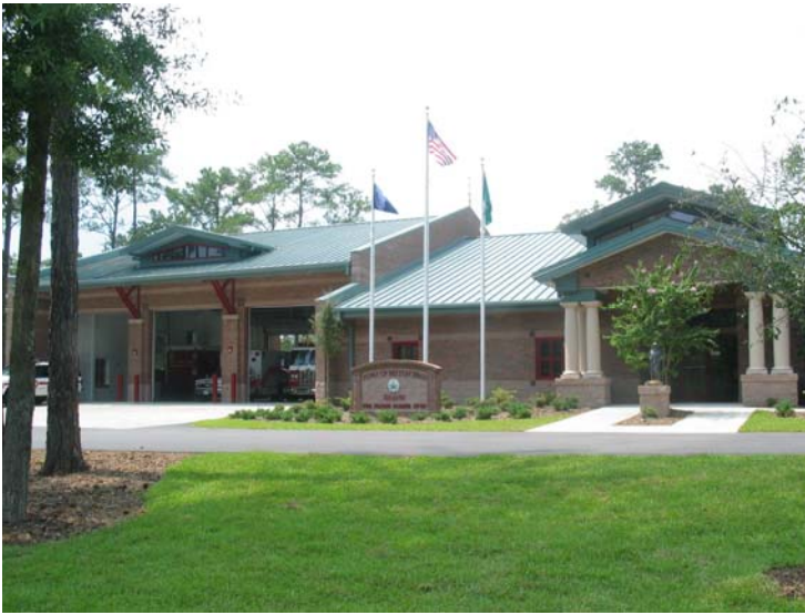
Hilton Head Island SubStation: Example of Pre-Engineered Construction
