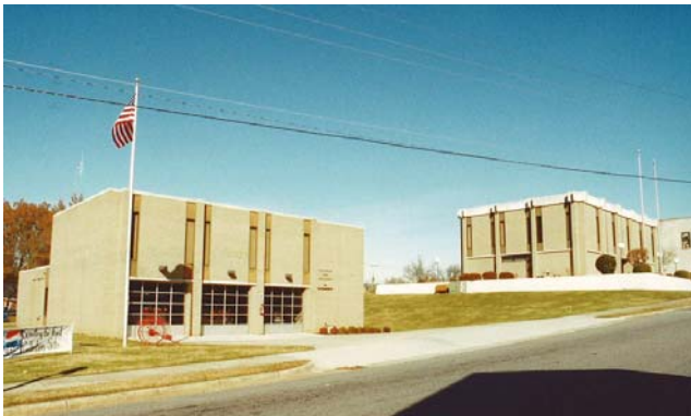
Lincolnnton Fire Dept & City Hall before renovations.
