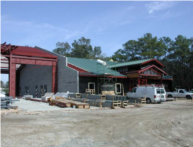
Hilton Head Island SubStation: Pre-Engineered Under Construction
