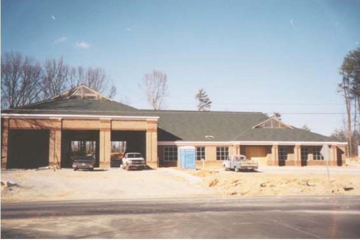
Conventional Construction During Construction
