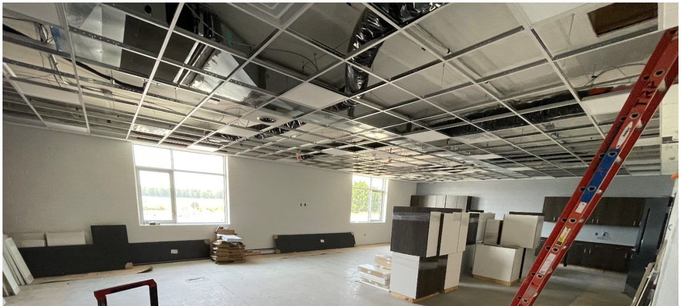
Training Room Ceiling Grid Installed
