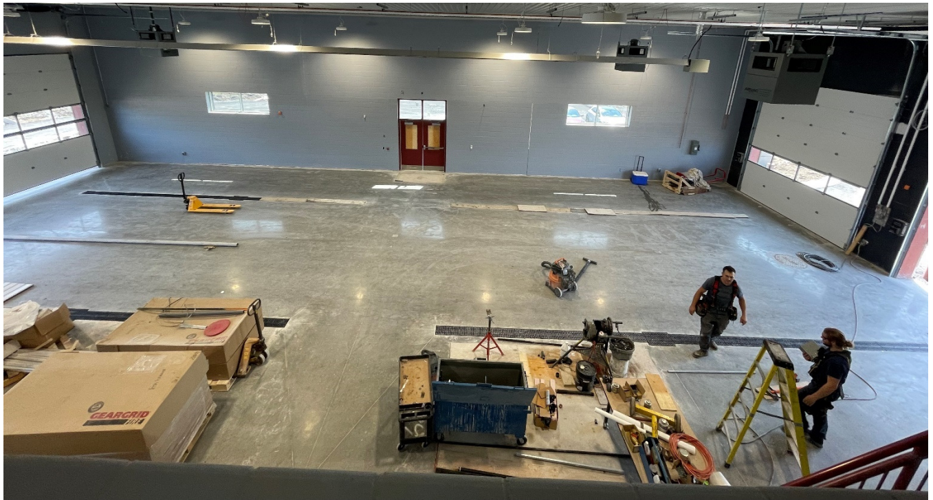
Apparatus Bay Floor Polished
