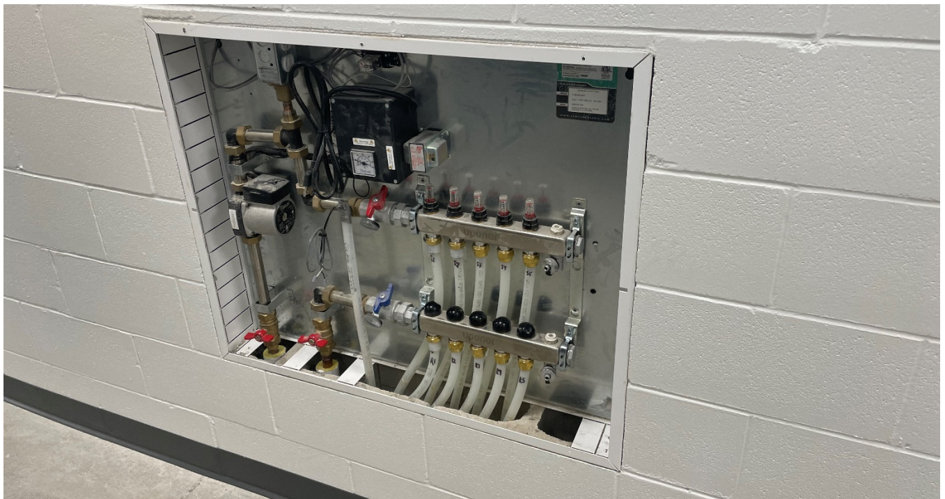
In-floor heating Manifolds Complete
