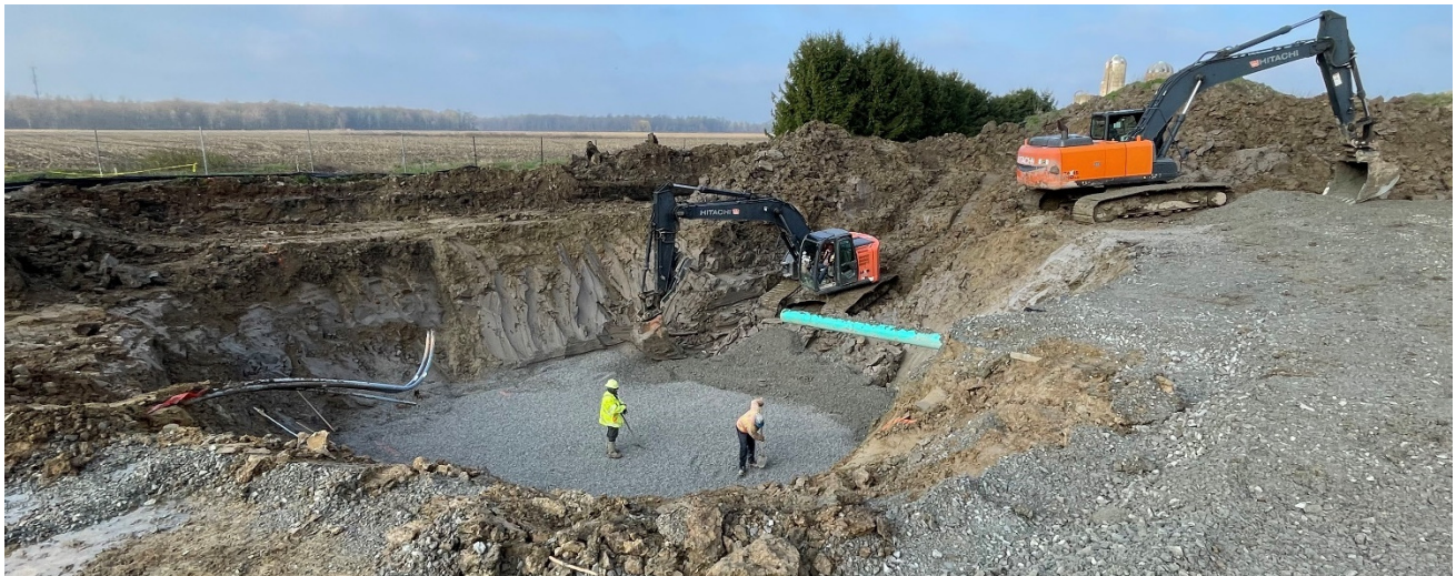
Excavation for Fire Cisterns
