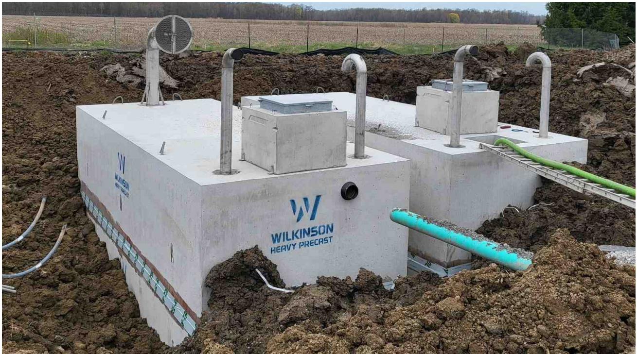
Fire Cisterns Installed
