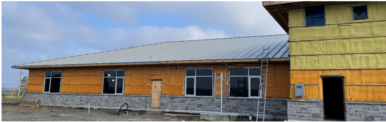
Metal Roof Installation – Brick Veneer complete
