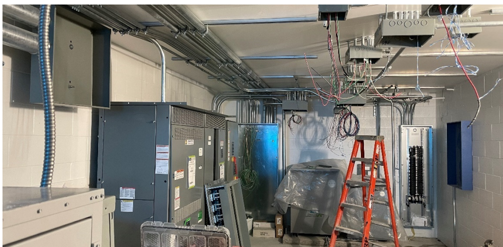
Mechanical Room Electrical Switchgear & Breaker Panels
