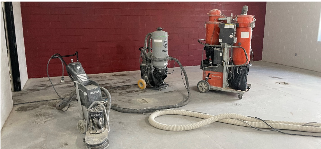
Floor Grinding & Polishing – Training Room
