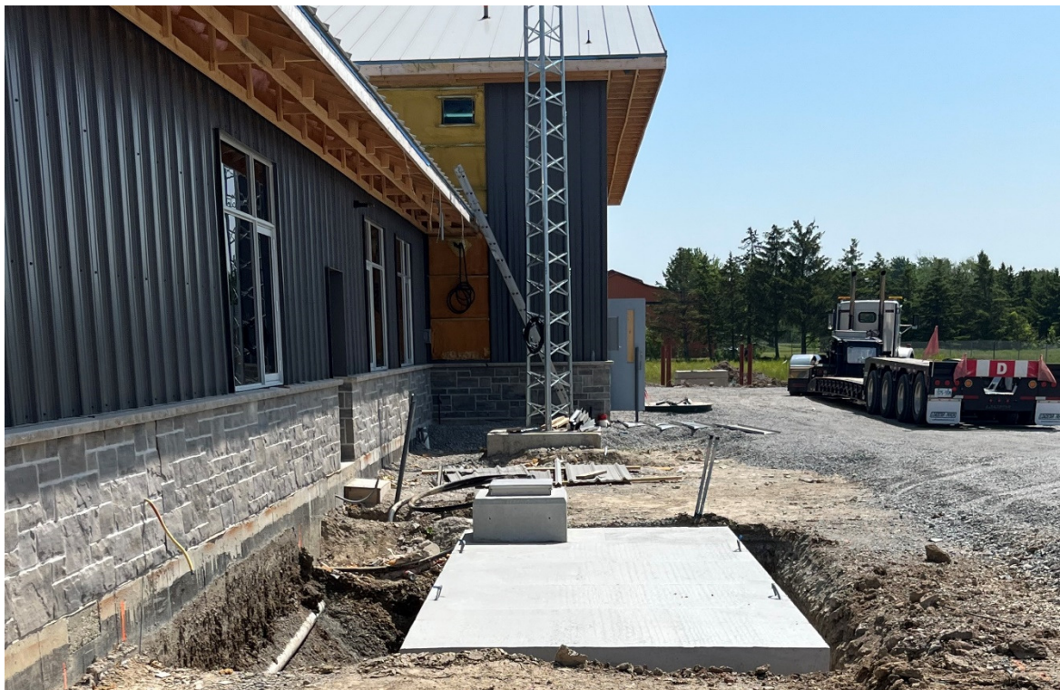
Potable Water Cistern Installed
