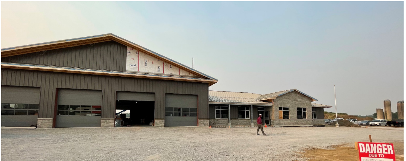
Roof, Apparatus Bay Doors Complete – Siding Installation
