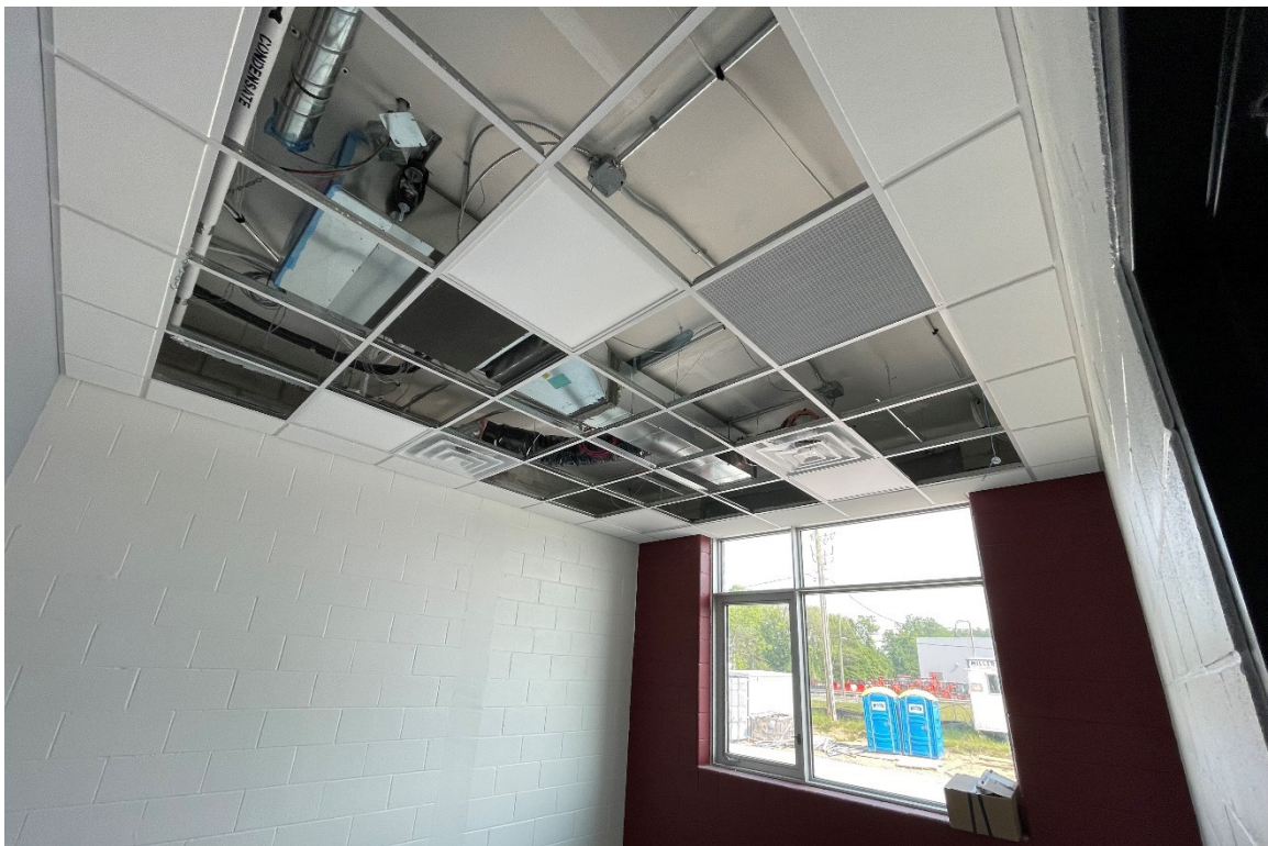
Ceiling Tile, Light Fixture, HVAC Diffusers Installation
