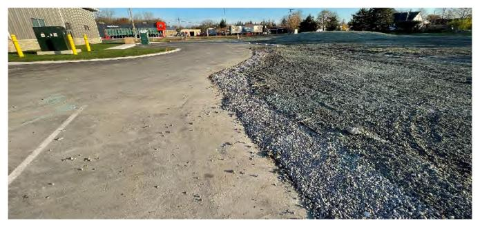
Road Base Sub-Drains Installed, Hydroseeding Complete
