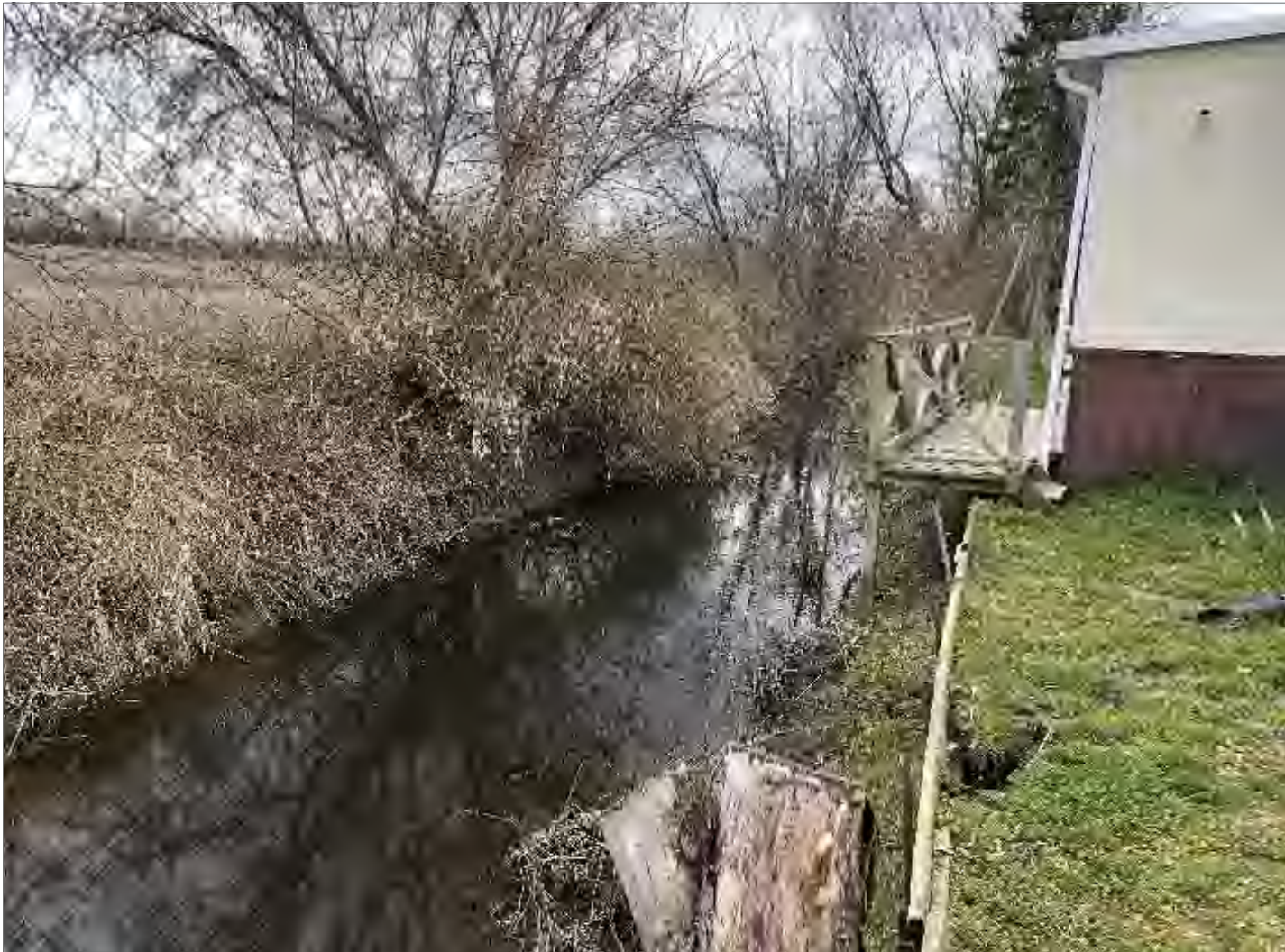
SITE PHOTO #1: PROXIMITY OF EXISTING BUILDING TO ELLSWORTH MUNICIPAL DRAIN (AS OBSERVED FROM NORTH BANK, LOOKING WEST) APRIL 16, 2020 (RJB)
