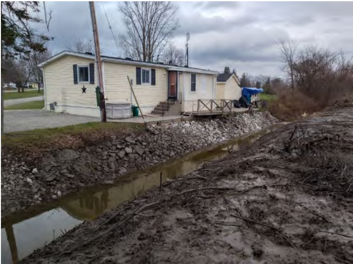
Figure 1: Temporary channel grading and erosion protection
