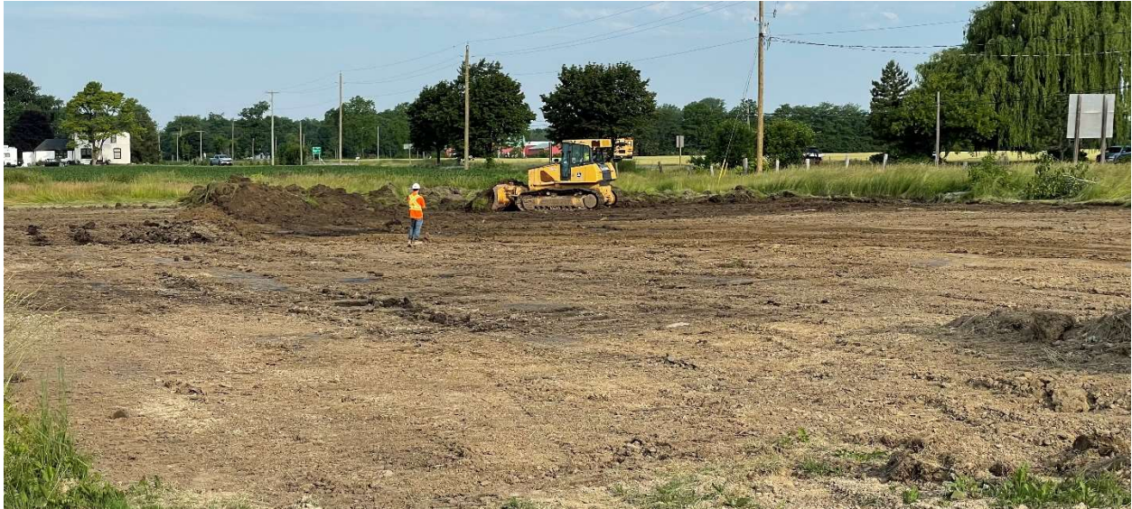
Stripping Topsoil
