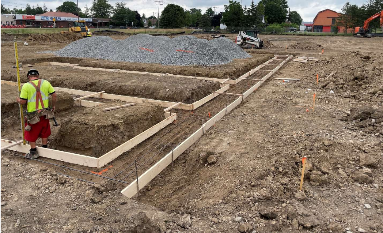
Forming and Reinforcing of Footings
