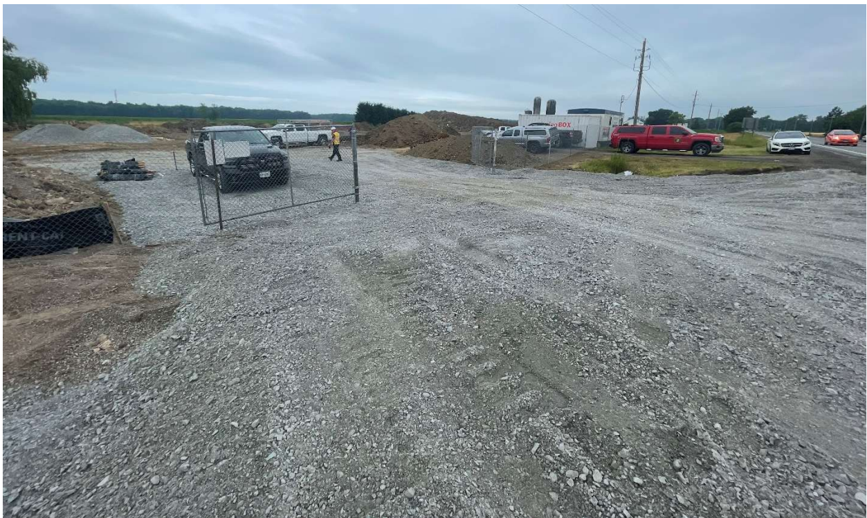
New Site Entrance Constructed
