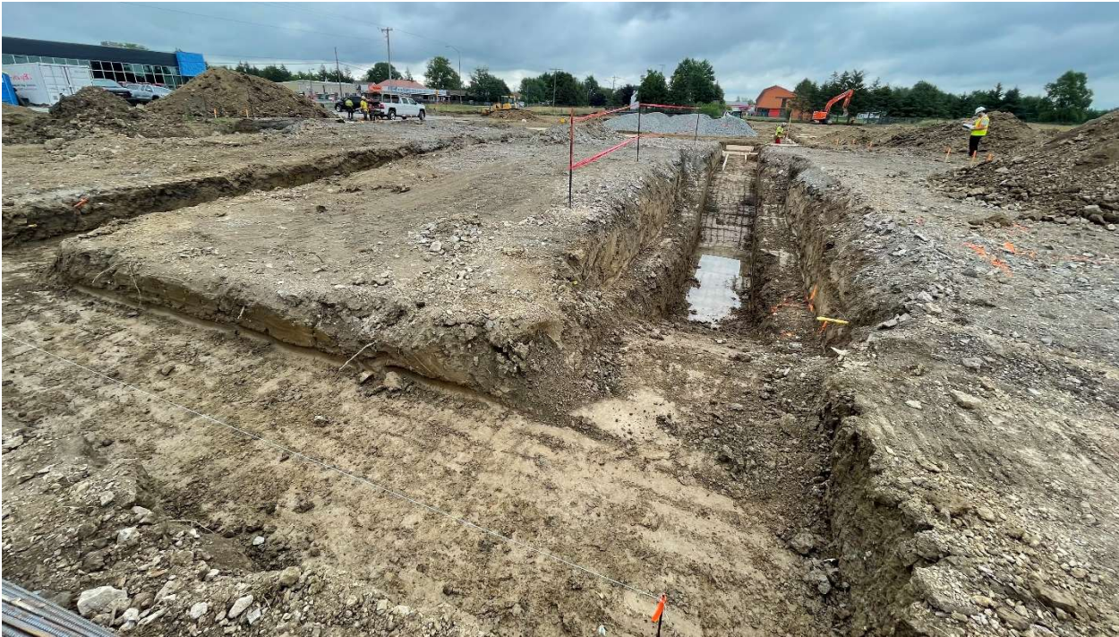
Excavation for Footings
