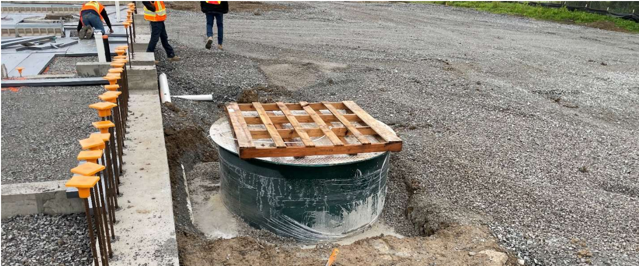
Extractor Tank Installed
