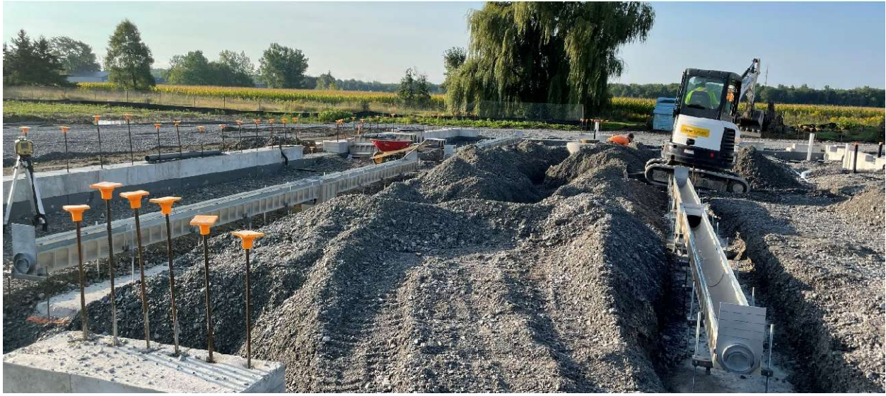
Apparatus Bay Trench Drain Installation
