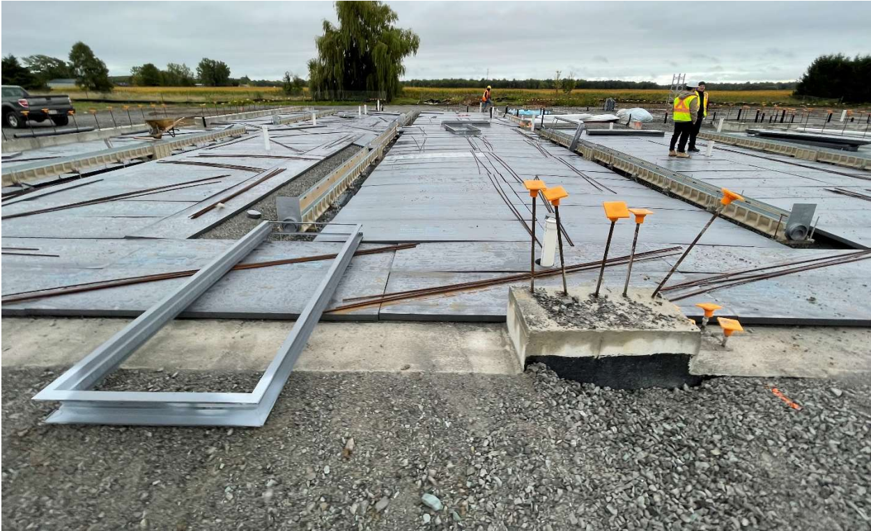
Under Slab Insulation Installation
