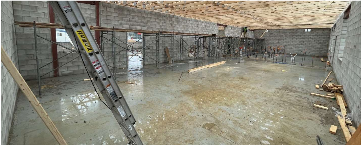
Administration Load Bearing Masonry Complete – Training Room
