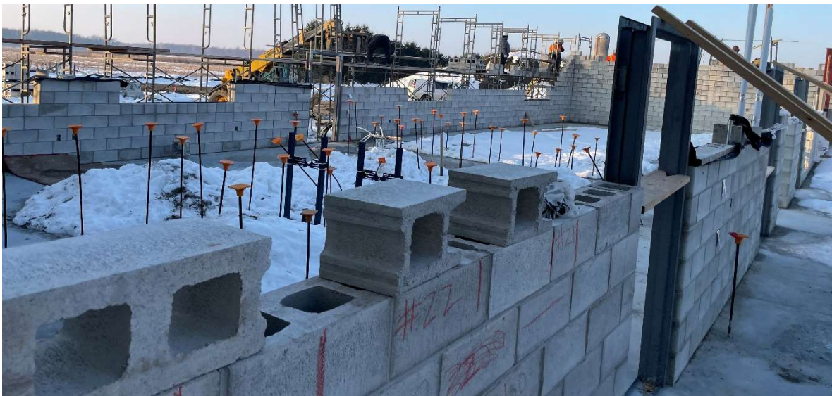
Administration Load Bearing Masonry Commenced
