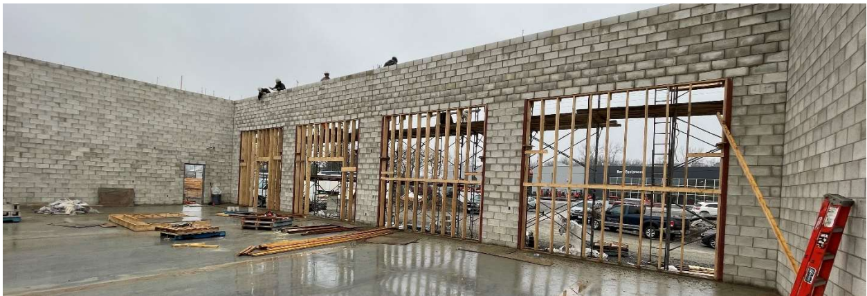
Apparatus Bay Masonry Exterior Complete
