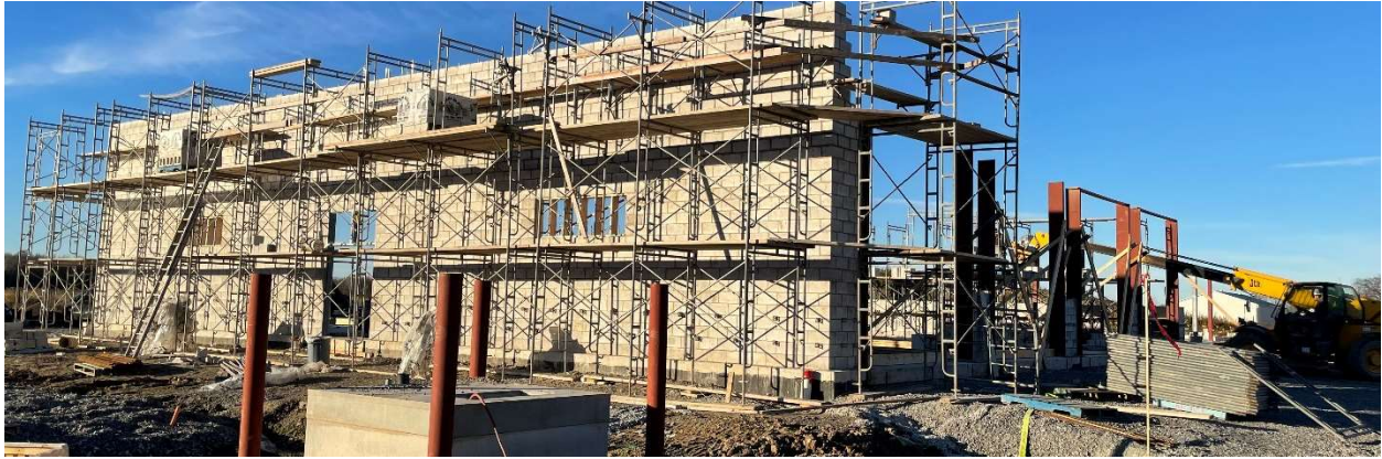
Apparatus Bay Masonry Commenced
