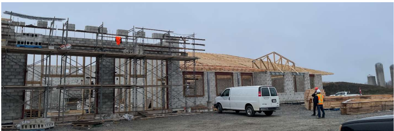
Roof Trusses Installed – Administration Area
