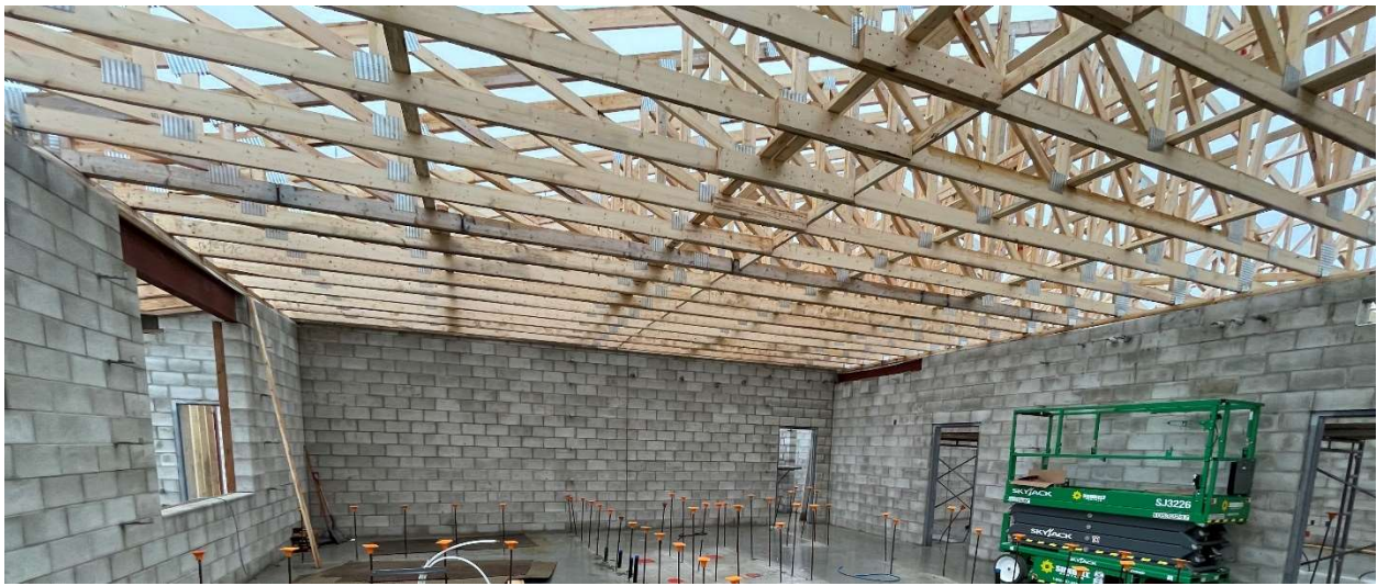
Roof Trusses Installed – Administration Area
