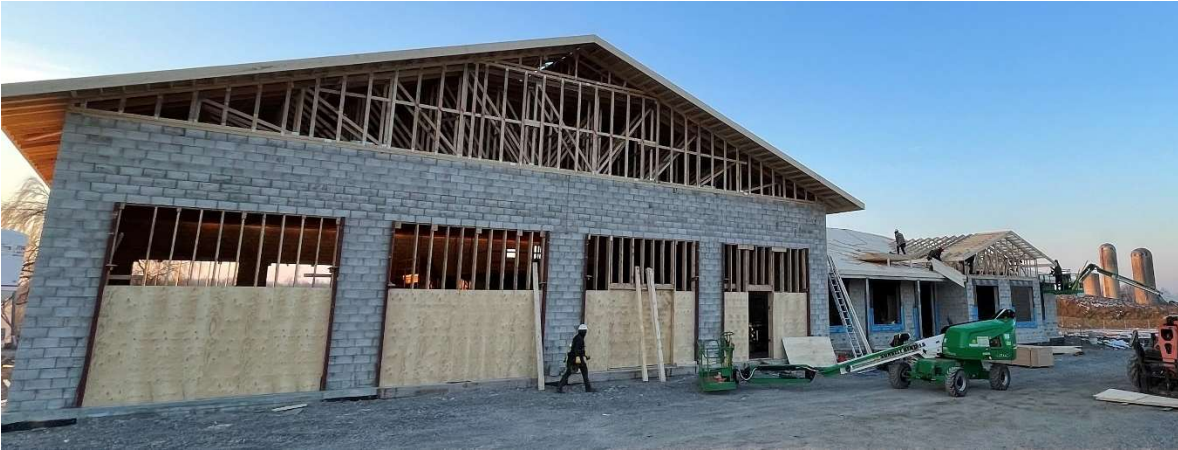
Roof Trusses & Sheathing
