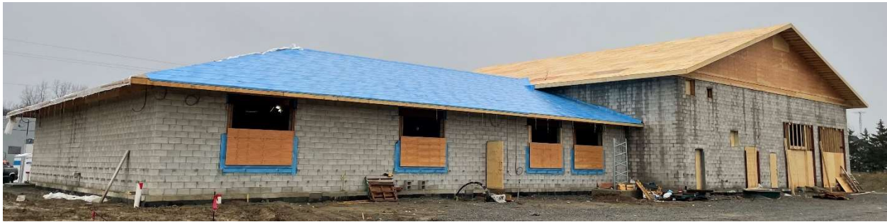
Roof Membrane Installed South Side of Administration
