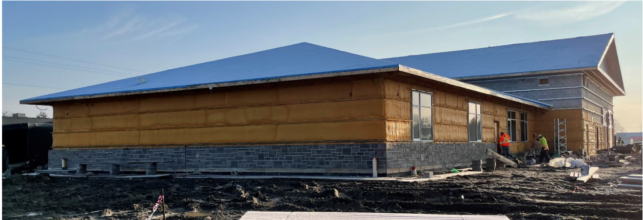
Brick Veneer Installation
