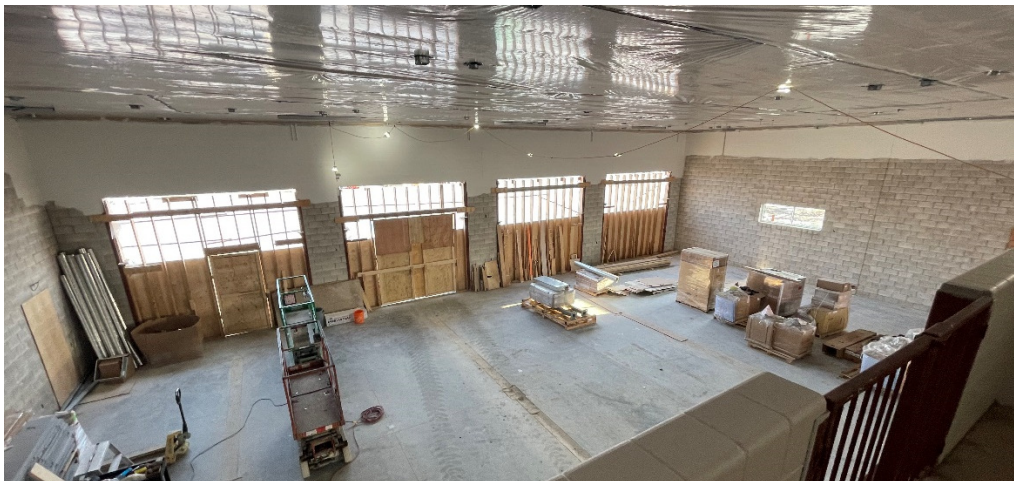
Apparatus Bay – Vapour Barrier Installed, Painting Commenced
