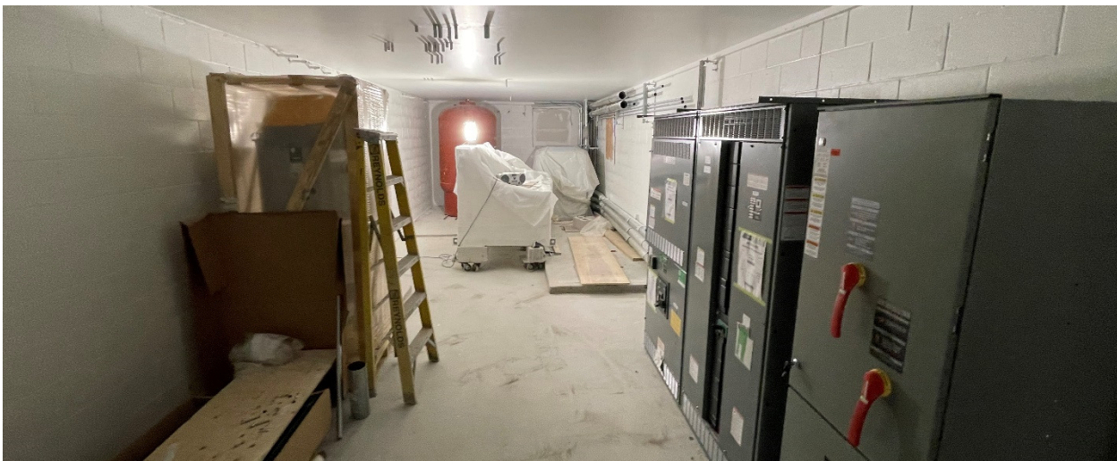
Mechanical Room- Painted, Switchgear installed
