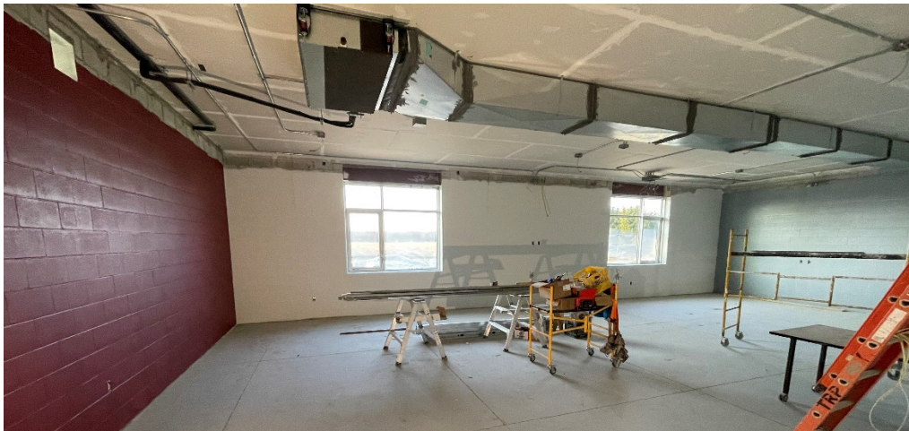
Training Room- Painted, Mechanical Equipment and Ductwork Installed
