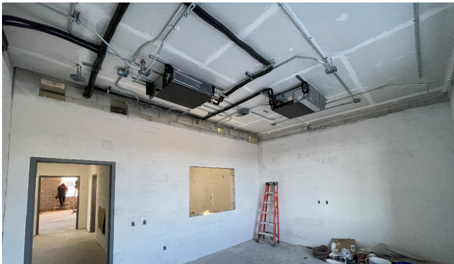
Kitchen – Primer, Mechanical & Electrical Equipment Installation
