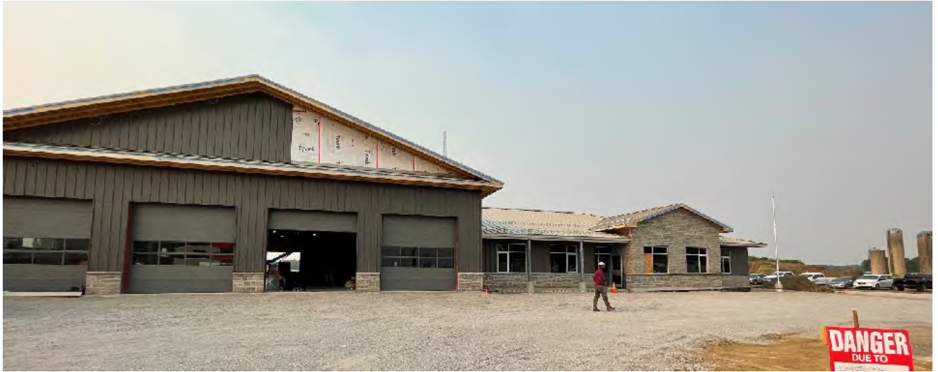
Roof, Apparatus Bay Doors Complete – Siding Installation
