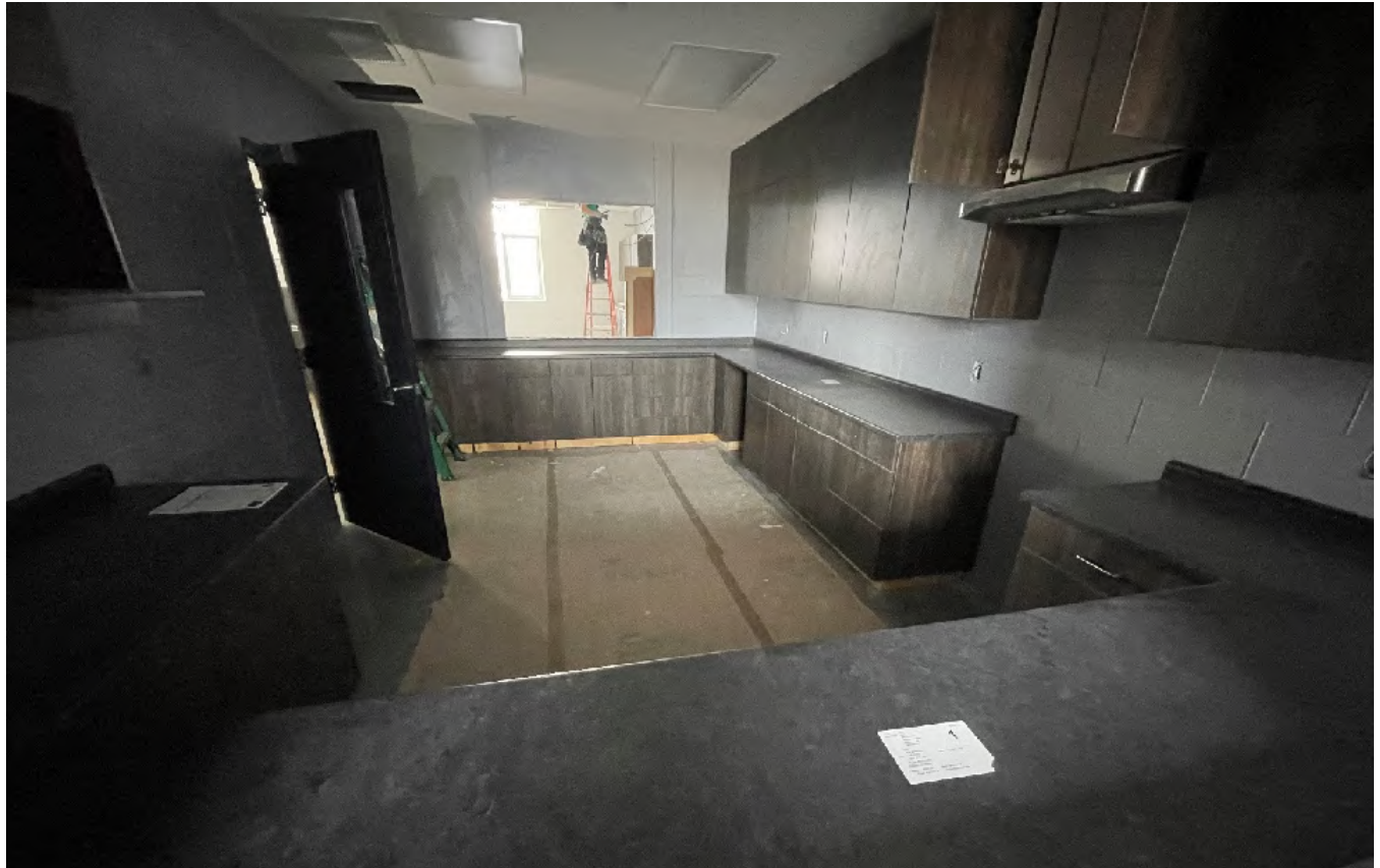
Kitchen Ceiling, lighting, Millwork and Counter's Complete
