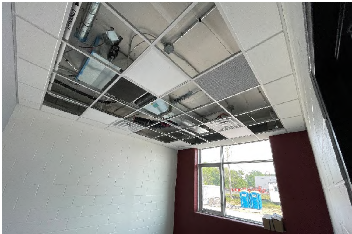
Ceiling Tile, Light Fixture, HVAC Diffusers Installation
