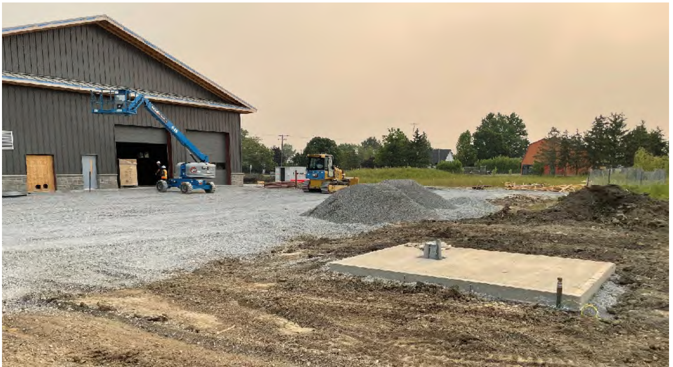
Generator Pad Poured
