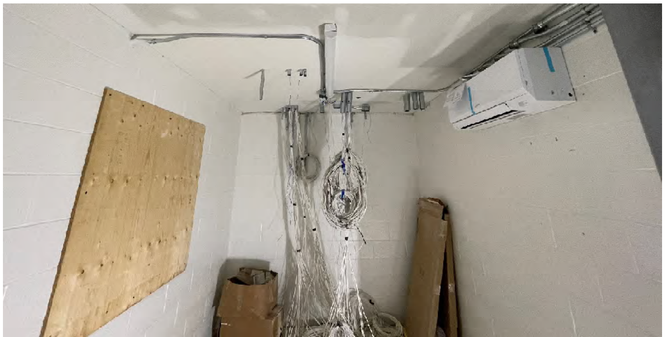
IT Room HVAC and Drywall Complete
