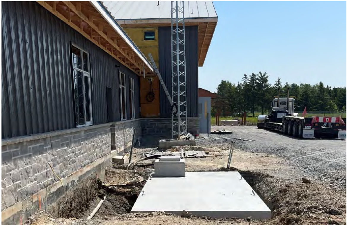
Potable Water Cistern Installed
