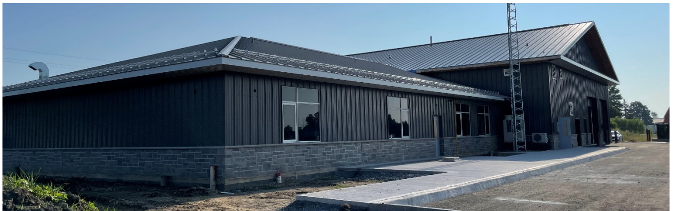
Siding, Soffit, Roof, Sidewalks, Curbs Complete
