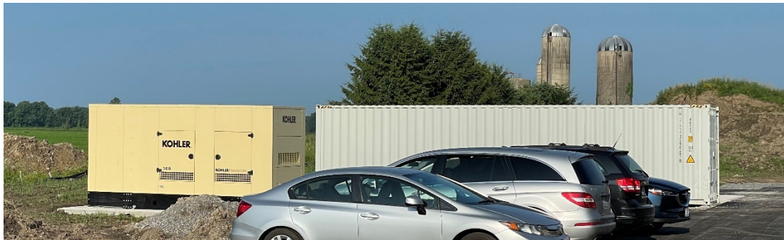
Generator Installed on Pad, Town Sea-Container Placed/Anchored
