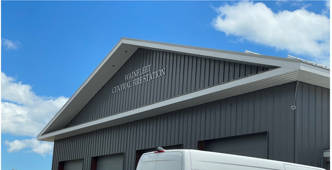
Siding, Soffit, Building Signage Complete at Apparatus Bay
