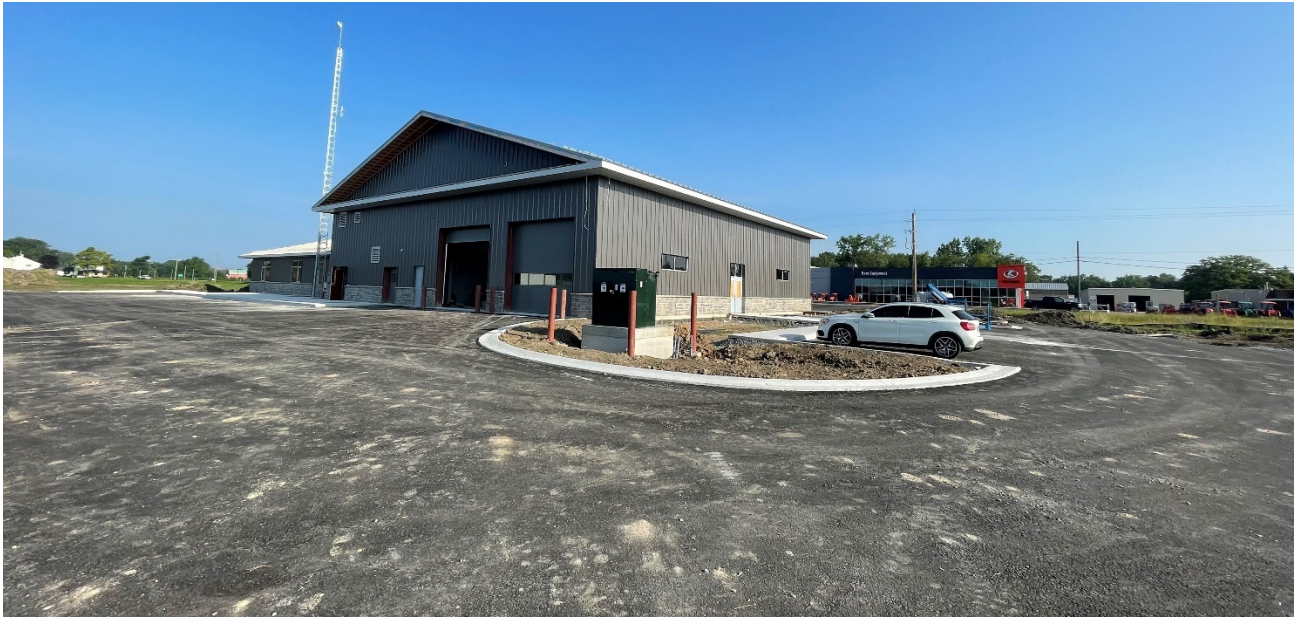
Curbs & Base Course Asphalt Complete
