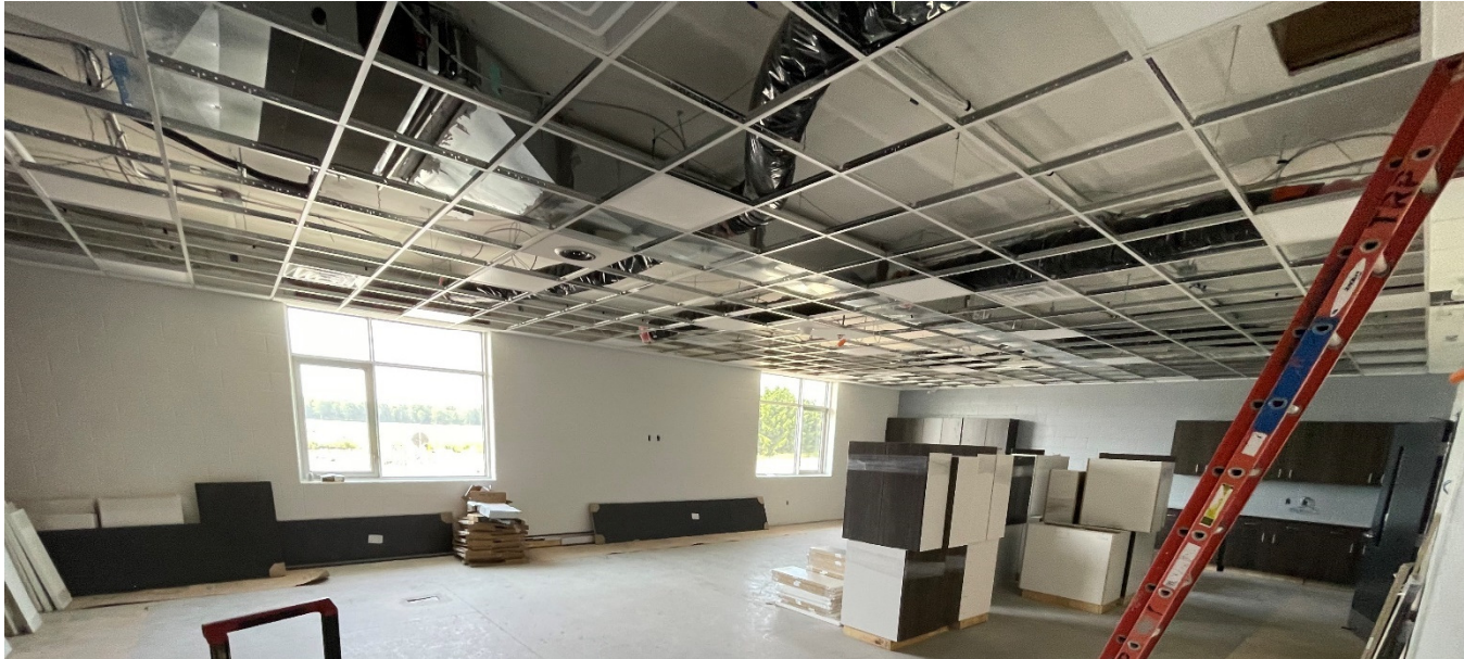
Training Room Ceiling Grid Installed
