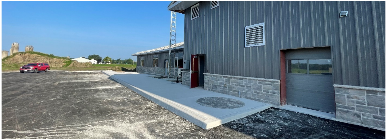
Concrete Sidewalks Complete
