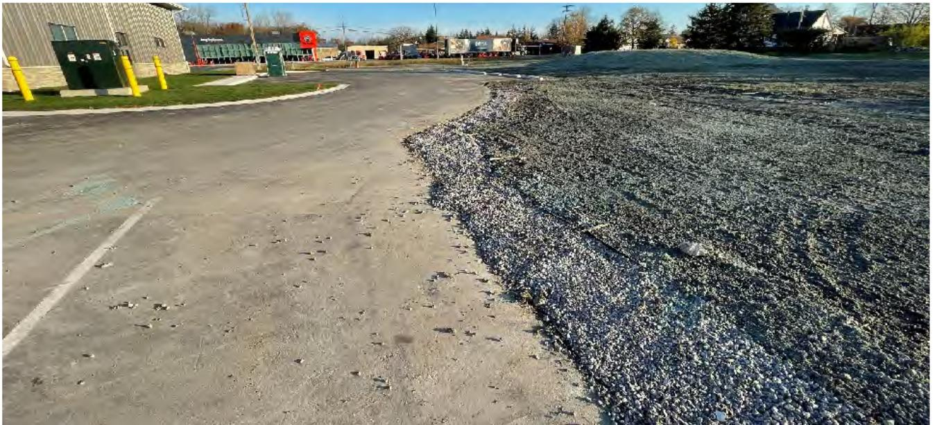
Road Base Sub-Drains Installed, Hydroseeding Complete
