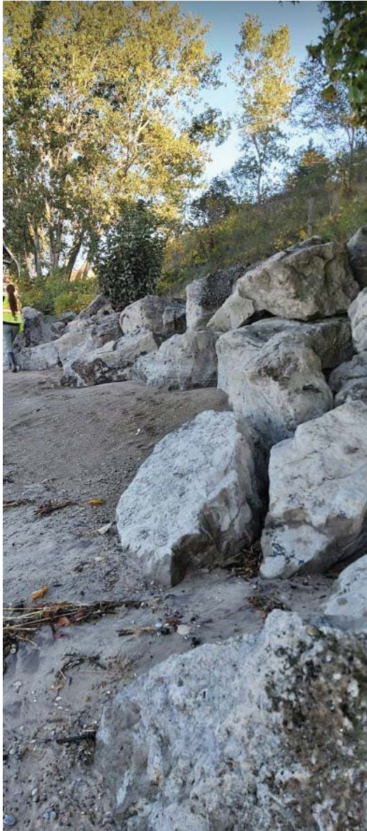
Toe of dune showing large armourstone, facing west
