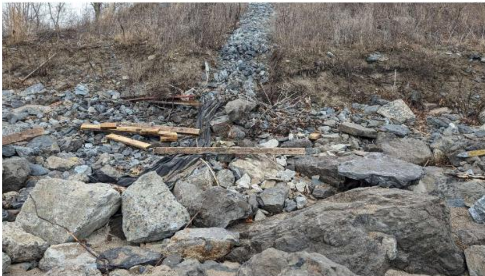
Figure 8 - Existing shoreline protection and drainage, looking north.
