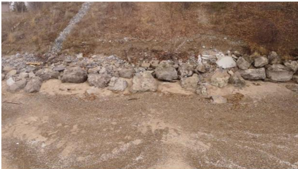
Figure 4 – Existing shoreline protection at the subject property.
