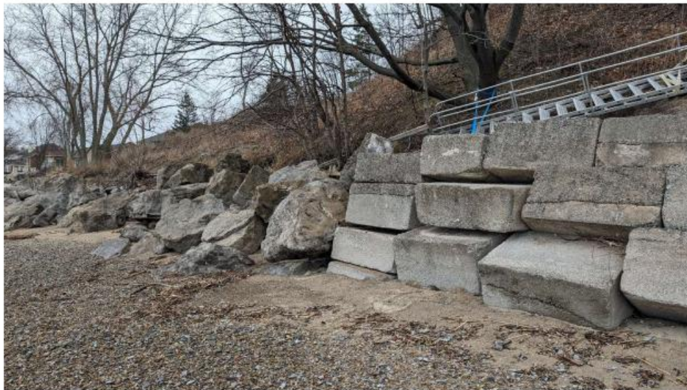
Figure 12 – Existing shoreline protection at the subject property, looking north-west.
