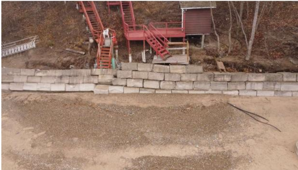
Figure 5 – Existing shoreline protection at the east neighbouring property.
