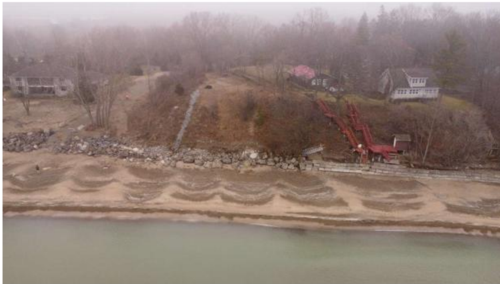
Figure 2 – Oblique aerial of the existing shoreline protection at the subject and east neighbouring properties, looking north.
