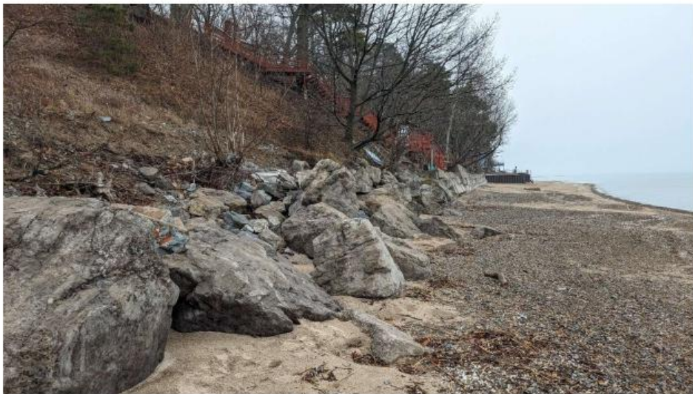
Figure 6 – Existing shoreline protection, looking east.
