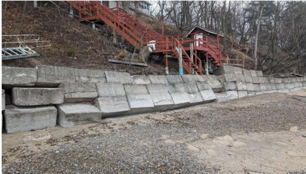
Figure 11 – Existing shoreline protection at the subject and east neighbouring property, looking north-east.
