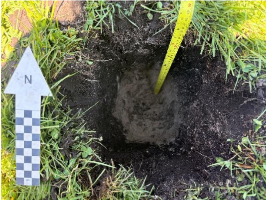
Image 17: Typical test pit with dark brown topsoil and yellow-brown subsoil.
